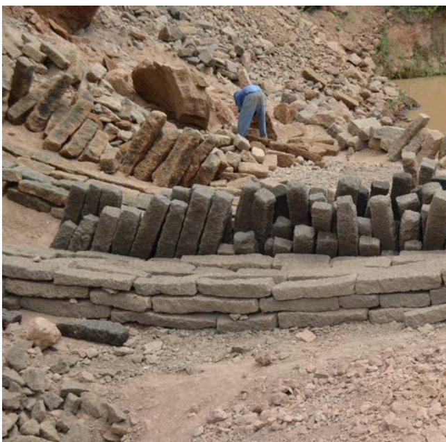
Ready Stone at Mutonga River Quarry
